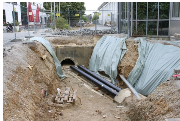
Figure 14: Construction of a district heating system in Germany (Source: Rutz)
