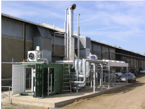
Figure 32: ORC system (using R245fa) of a biogas plant in Dublovice, Czech Republic (Source: GE Energy)
