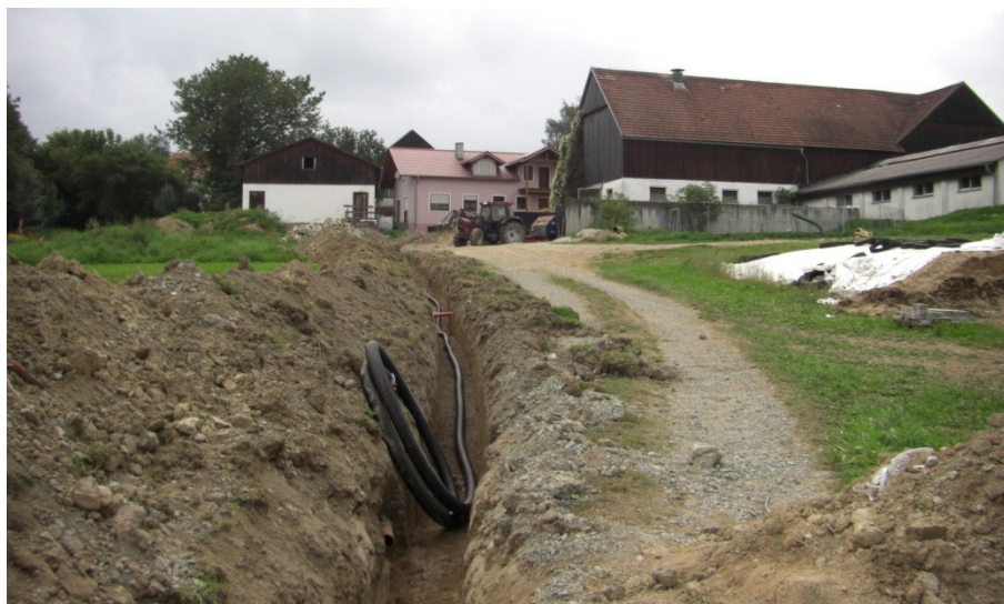
Figure 12: Installation of a heat pipe to the buildings of a farm (Source: Thermaflex Isolierprodukte GmbH)
