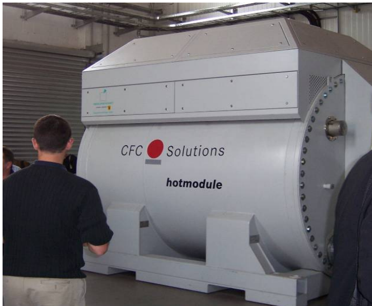
Figure 3: Molten Carbonate Fuel Cell (MCFC) for biogas in Leonberg, Germany (Source: Rutz)
