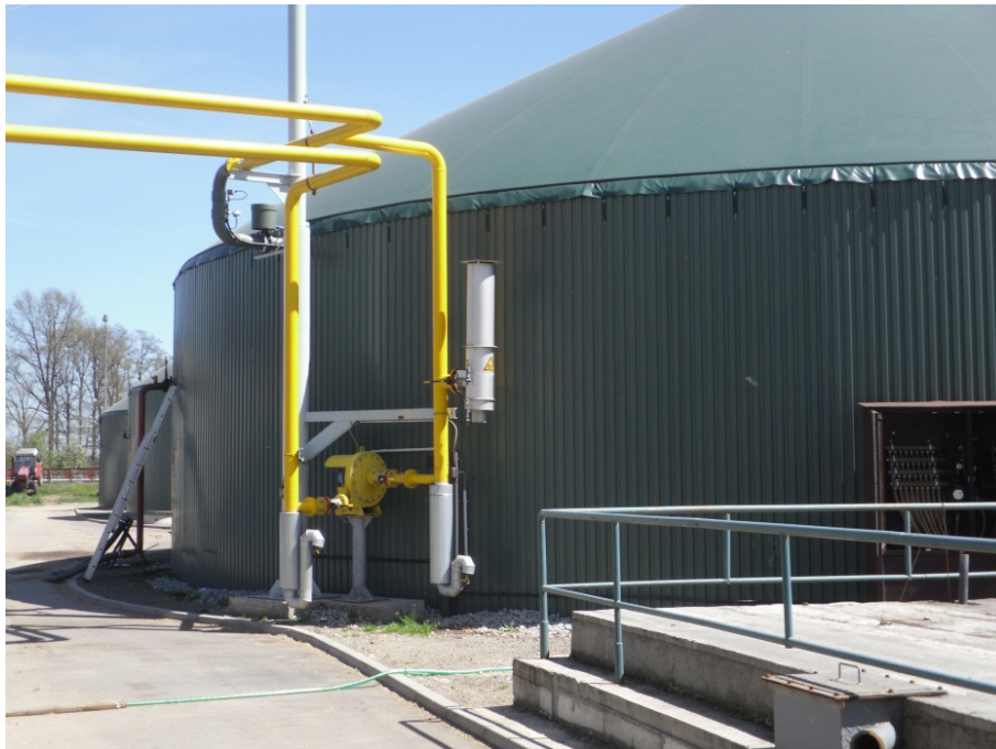
Figure 39: Start of biogas pipes to a satellite CHP unit to the town of Trebon, Czech Republic (Source: D. Rutz)
