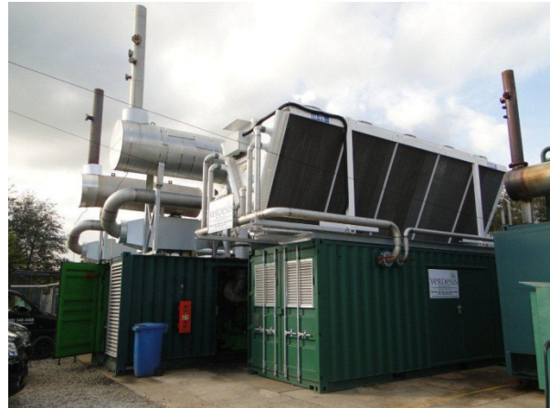
Figure 33: ORC system (using R245fa) (container in the front) and biogas engines (container in the back) of a landfill site in Warrington, U.K. (Source: Verdesis Services UK Limited)
